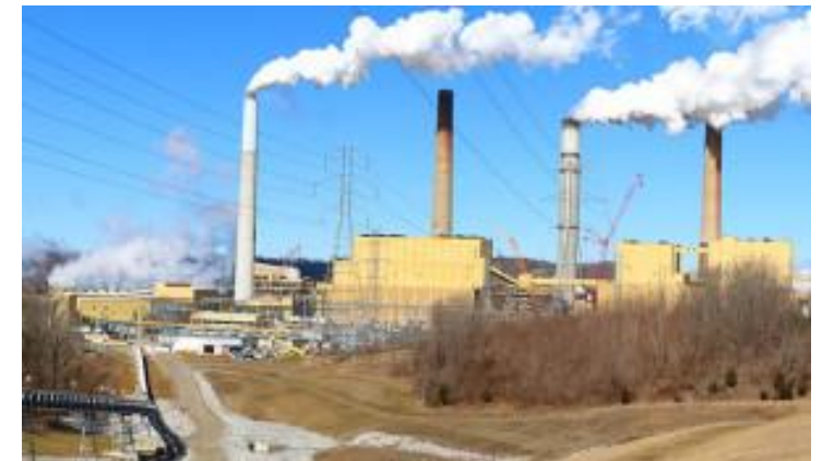
Ghent Generating Station Owned/Operated by Louisville Gas and Electric Company and Kentucky Utilities Company Located in Carroll County, KY
