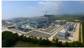
HTR-PM, China 2x110 MWe HTGR Under Commissioning
