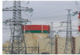
Ostrovets 1 - Belarus VVER V-491 In operation
